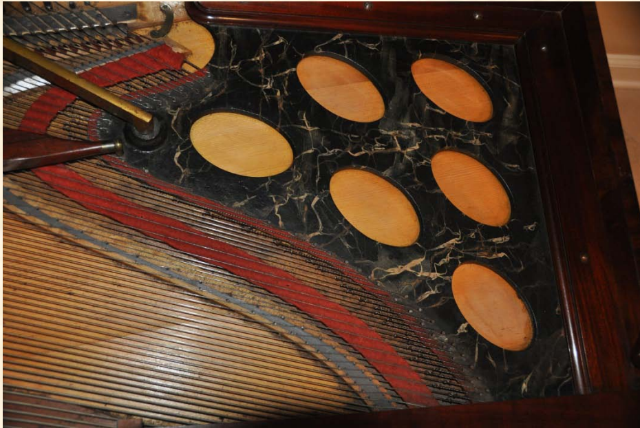
String plate w/ unichord stringing. Given the tension required for these strings, a metal hitch pin plate is necessary to prevent the pin being ripped from its seat.
